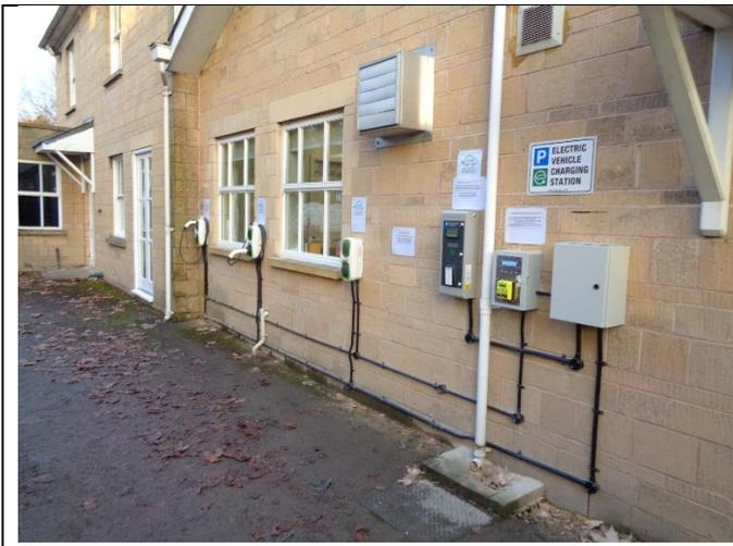
The contactless card car charge points in Monmouth with 3kW, 7kW and 20 kW type 1 and type 2 cables
